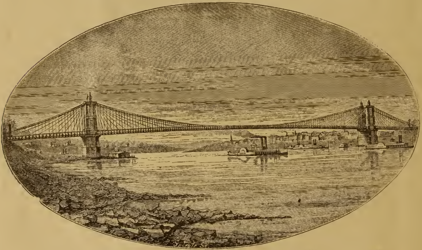
Covington and Cincinnati Suspension Bridge, built by JOHN A. ROEBLING. Main Span, 1,057 feet.
